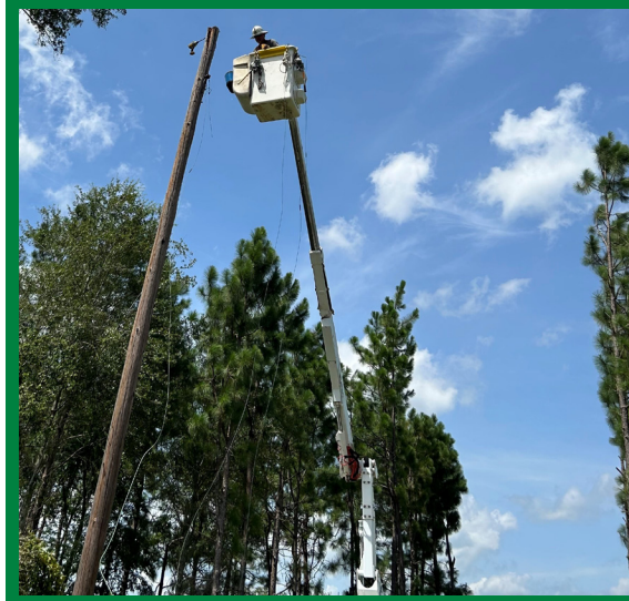
Excelsior EMC Crew Leader, Jamey Donaldson, booms up to the top of a damaged pole to make repairs after falling trees tore down the wire.
