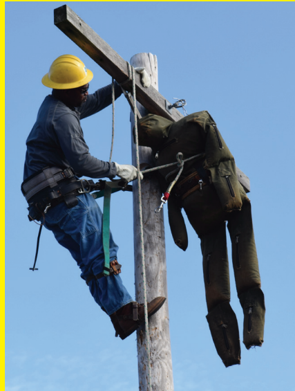
Lineman Micheal Byrd practices a pole top rescue during a monthly employee safety meeting.
