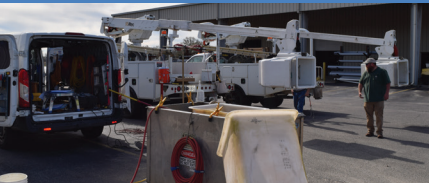
Technicians conduct a visual inspection of the truck's boom components before testing.
